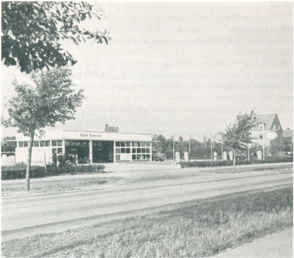
Moderne service station (Esso).
