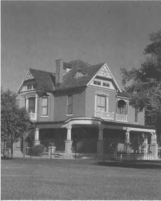
Petersen House Museum i Tempe i Arizona.
