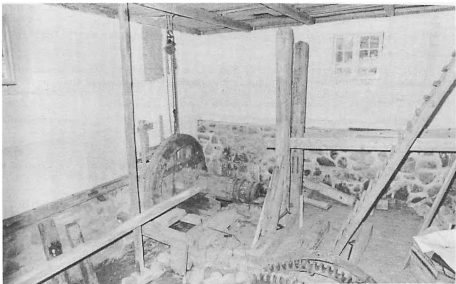
Fig. 17: neg. 1726.03: 06-08-64: Monteringen af maskineriet begyndt. Erecting the milling plant has commenced.
