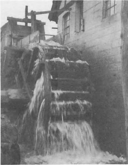
Fig. 32: neg. 17.05: 31-03-39: Vandhjulet igang i Svanninge . . . . . Waterwheel working in Svanninge . . . . .
