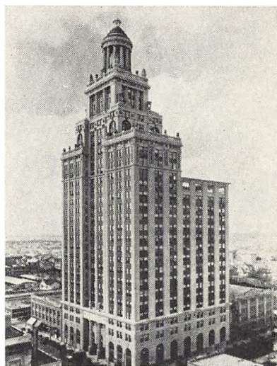
The Esperson Bldg. i Houston, Texas
