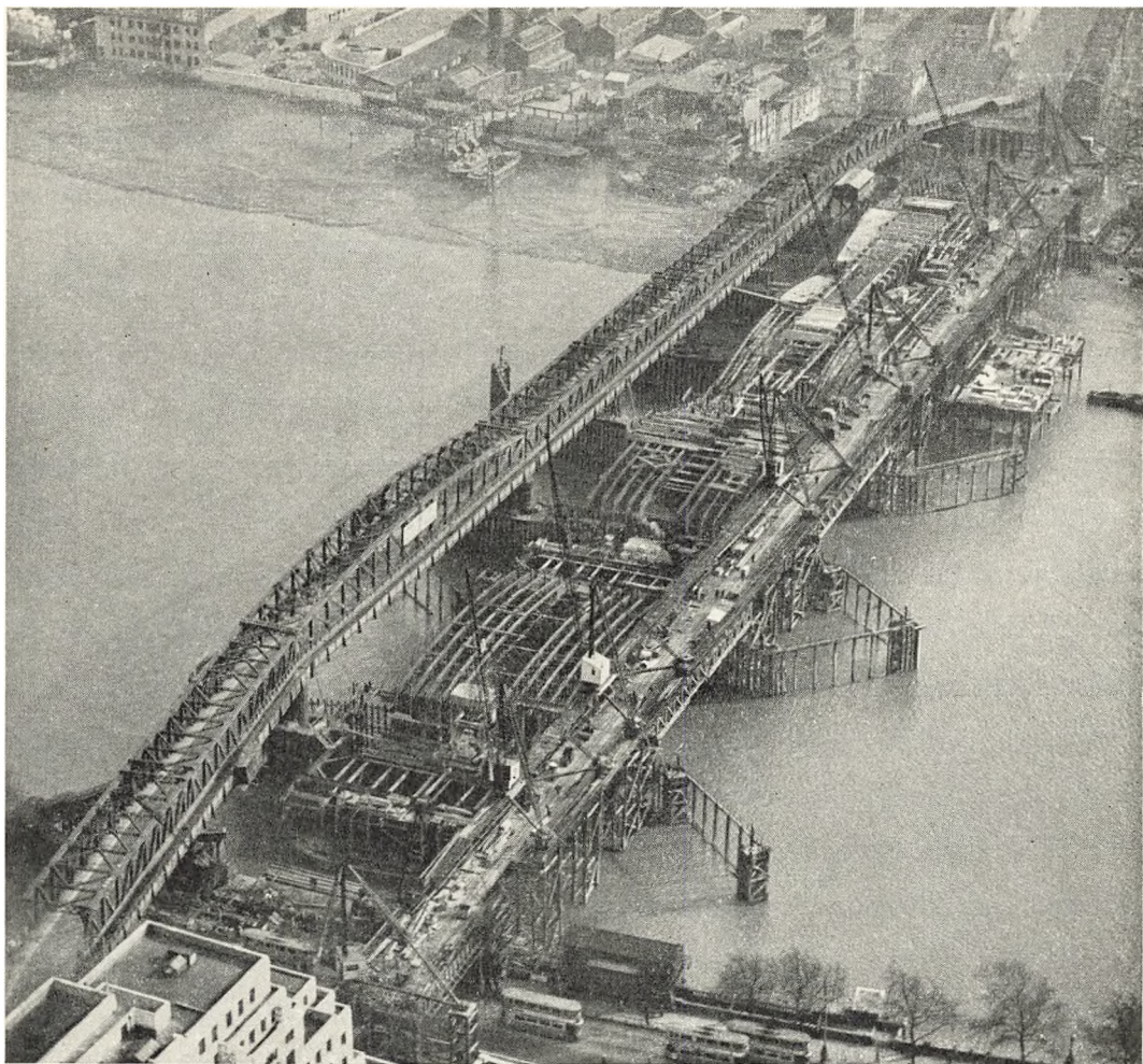
Den ny Waterloo Bridge under Bygning
