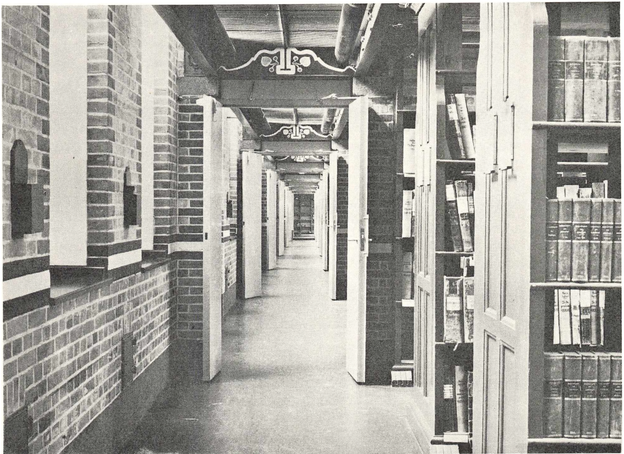
Glimpse of one of the long corridors in the Nyrop building of the Provincial Archives of Sealand. In connexion with the rebuilding fire doors were put up between the various sections.
