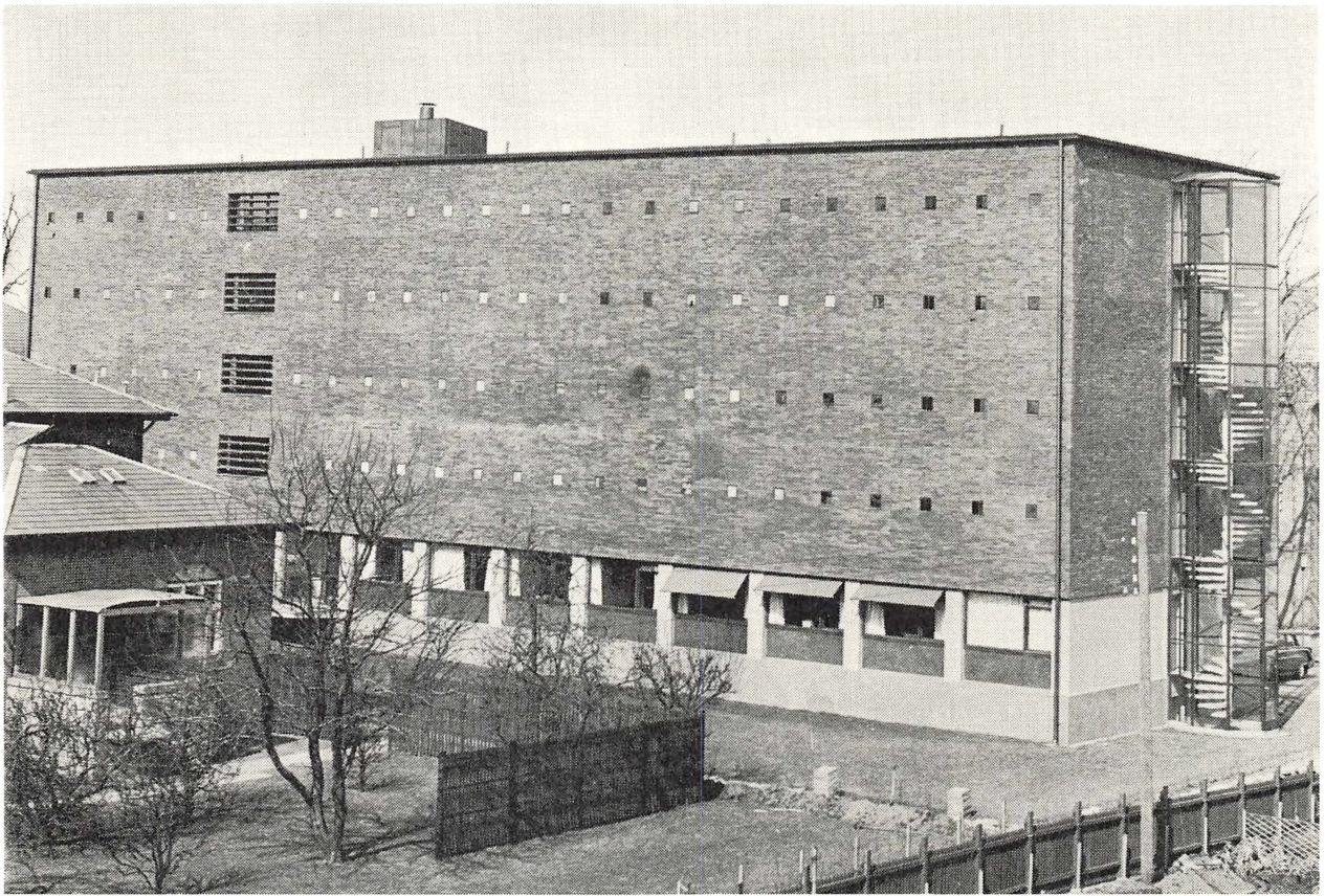
The new depot of the Provincial Archives of North Jutland with the stair turret.
