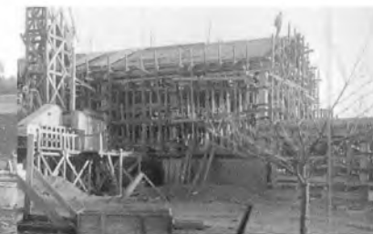
Filterbygningen tager form.
