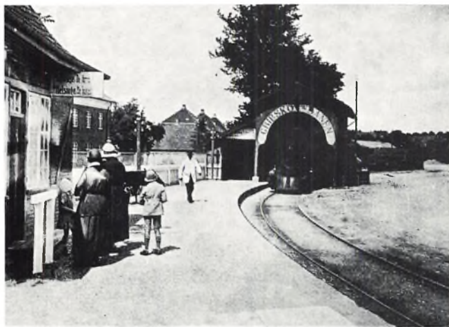
Gribskovbanens station i Hillerød 1905.
