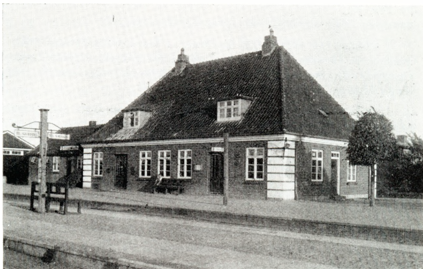
Øster Vraa Jernbanestation.
