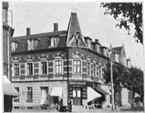
22. Øster Boulevard 13, dateret 1902.
